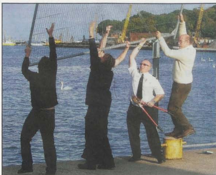
■ Drastic action – a section of the fence had to be removed
